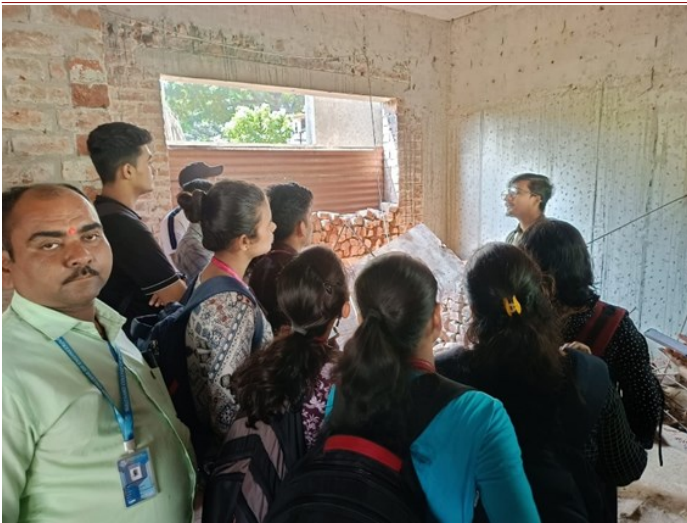
Site Visit at PWD Guest house-II, Sangli Saturday 7 th Oct., 2023, Site Visit at Residential Building of Mr. Anand Shah, Sangli Saturday, 7 th Oct., 2023
