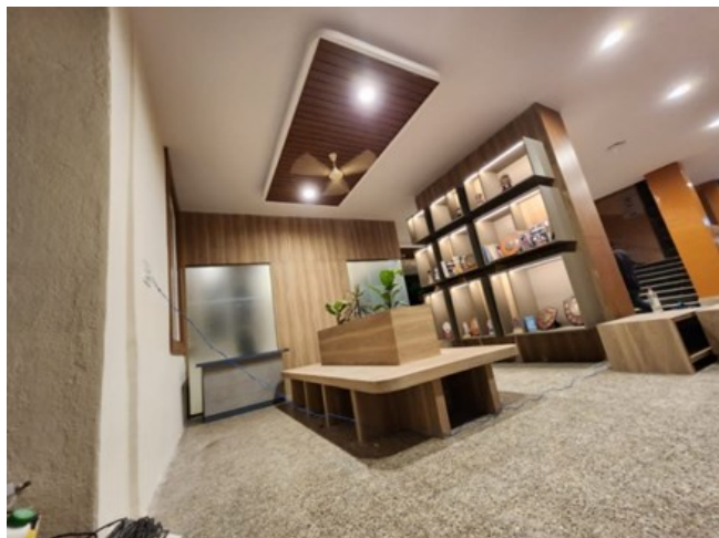
Renovation of Waiting area for Director Office in December 2023
