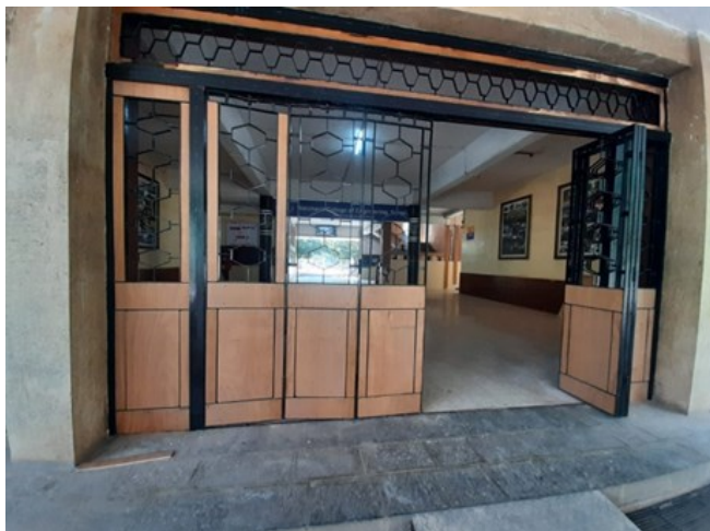
Repairs of Entrance Door in December 2023
